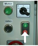
**8.** Press the **RESET** (green 1) button to put the pump into operable mode.
